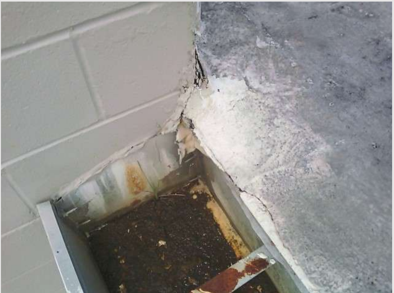
EXAMPLE OF EDGE FAILURE - LOSS
