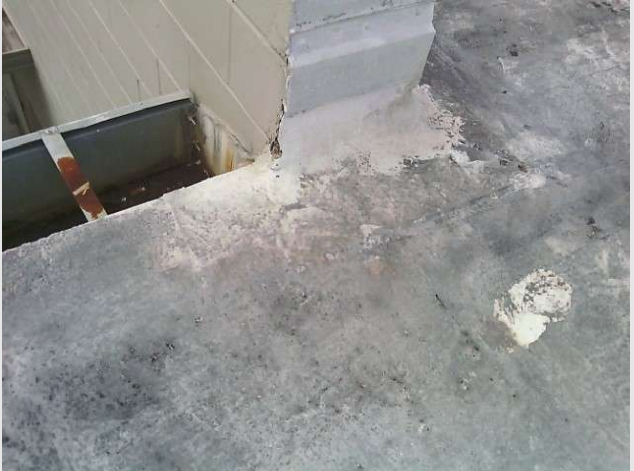
EXAMPLE OF EDGE FAILURE - LOSS
